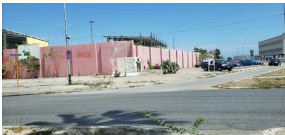
Current situation wall of former 'Coney Island'
