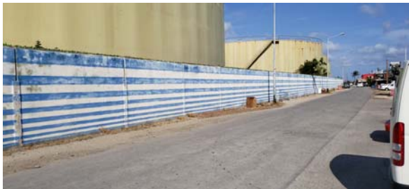
Current situation wall Aqualectra terrain
