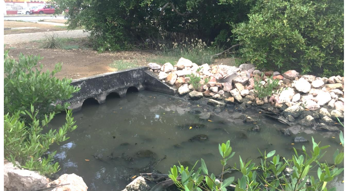
Sewage problem in mangrove area
